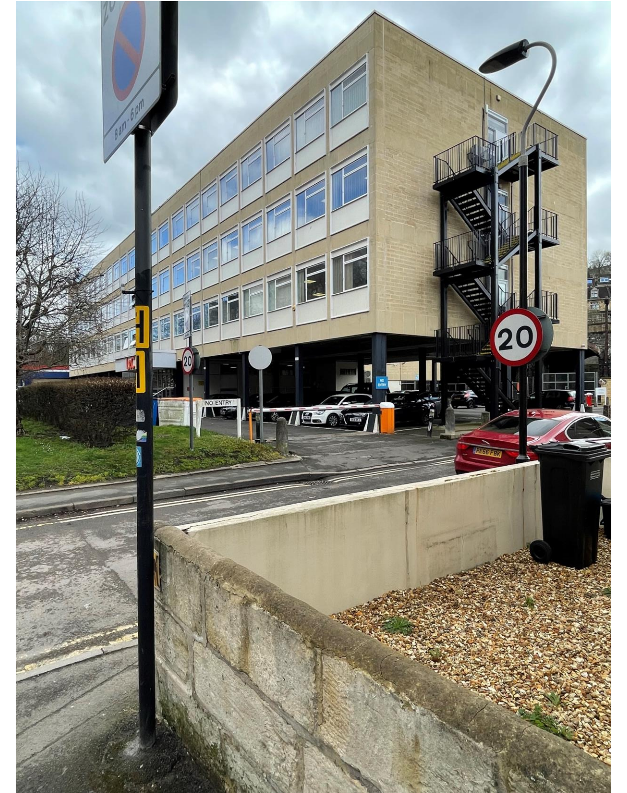
above: Beazer House at Oak Street and Lower Bristol Road
